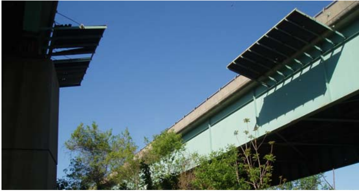
Figure 3. The I-476 bridge.
