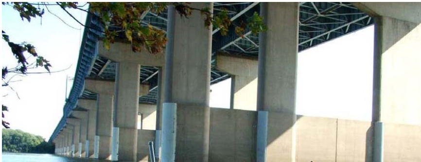
Figure 4. The I-81 bridge.
